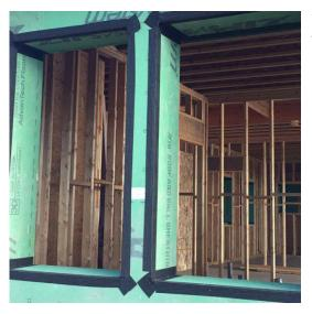
The black, fleece-backed flashing tape Fentrim F is the ideal flashing solution for jobsite conditions where mixed substrates are present.
